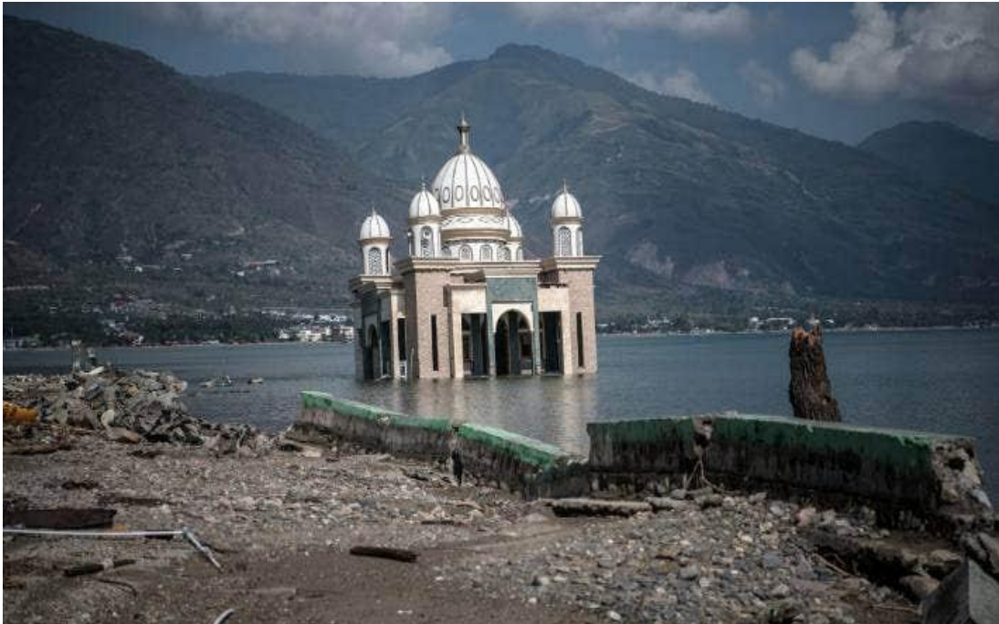
1-photo A mosque that was previously partially submerged sits at an angle after it was knocked off its foundations by an earthquake and a tsunami in Sulawesi.
